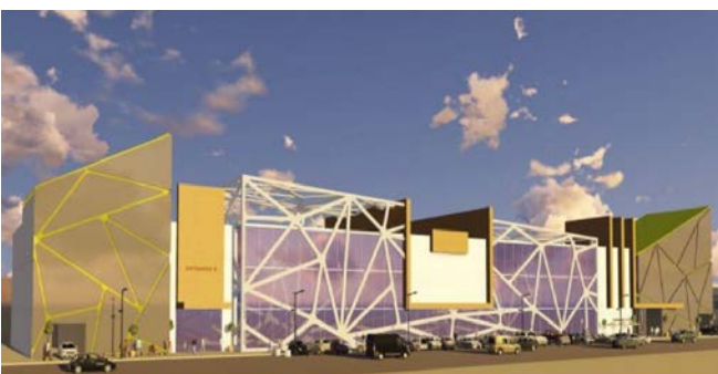
PROJECT: Mankhol Mall. My Role: Design and Supervision of Electrical Systems
