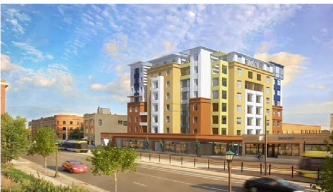
PROJECT: G+7+R Res / Com Building. Client: SHAIKH AHMED KHALIFA SAEED ALMAKTOUM Cost: AED 60 Millions My Role: Design and Supervision of Electrical Systems
