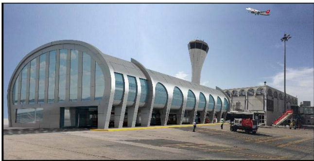
Sharjah International Airport Expansion Project Client: Sharjah Airport Authority Cost: AED 150 Millions My Role: Design and Supervision of Electrical Systems
