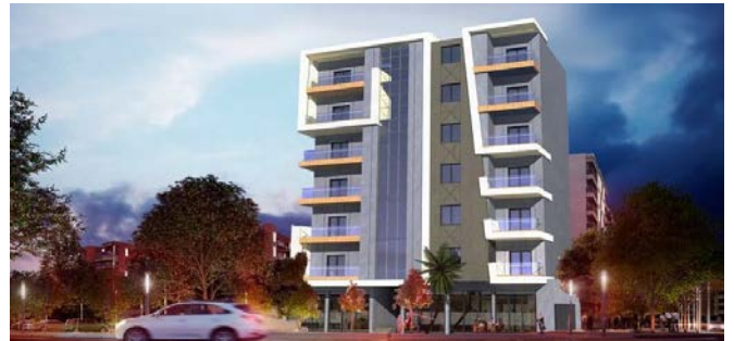
PROJECT: G+6+R Res / Com Building Client: SHAIKH AHMED KHALIFA SAEED ALMAKTOUM Cost: AED 20 Millions My Role: Design and Supervision of Electrical Systems
