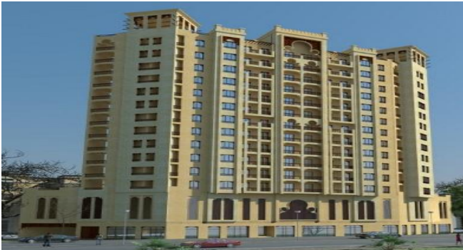
PROJECT: G+2P+12+R Res / Com Building Client: SHAIKH AHMED KHALIFA SAEED ALMAKTOUM Cost: AED 120 Millions My Role: Design and Supervision of Electrical Systems
