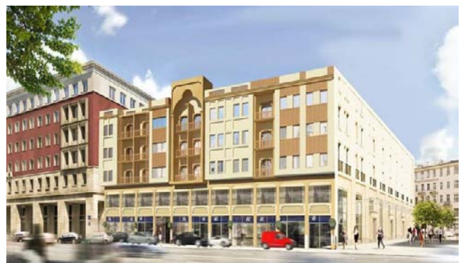
PROJECT: B+G+4+R Res / Com Building Client: SHEIKH HASHER BIN HAMAD ALMAKTOUM Cost: AED 70 Millions My Role: Design and Supervision of Electrical Systems
